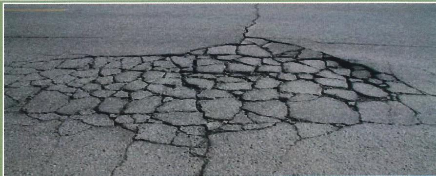
This condition is characterized by a series of interconnecting cracks that divide the pavement into many-sided, sharp-angled pieces resembling an alligator's hide. Alligator cracking usually occurs in wheel paths or other areas subjected to loading. Alligator cracking can be caused by weakness in the base or sub-grade, which results in the fatigue failure of the asphalt concrete surface under repeated loading.
