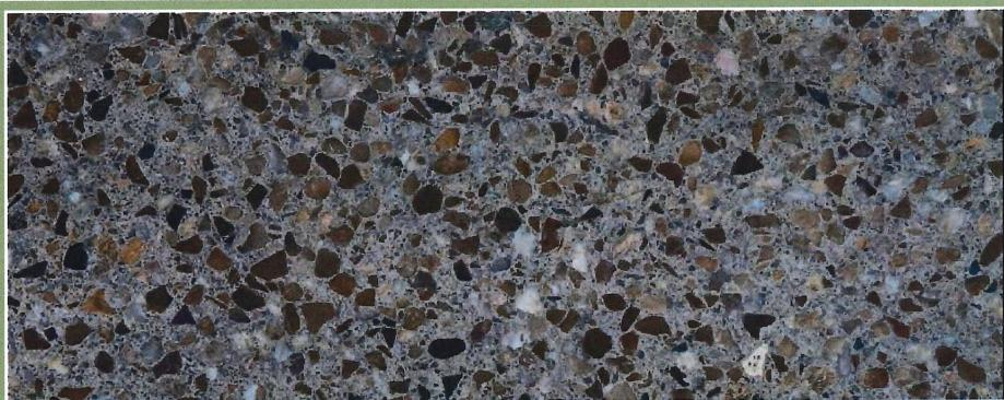
This condition is characterized by the wearing away of the pavement surface caused by the dislodging of aggregate particles and loss of asphalt binder. The pavement surface becomes smooth and rounded (and subsequently slippery) under the action of traffic. Polishing is normally caused by oxidation of the asphalt binder of the mix, resulting in loss of flexibility and ability to hold the aggregate.
