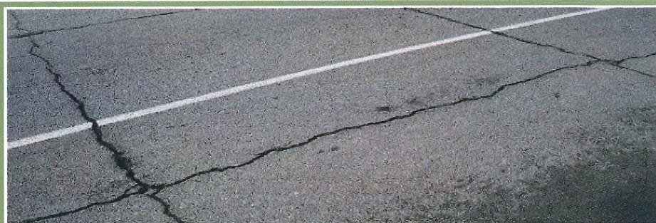
This condition is characterized by visible fractures or separations of the pavement surface occurring transversely across or longitudinally down the roadway. This cracking may be caused by a poorly constructed paving joint, shrinkage of the surface due to low temperature, asphalt hardening, or a reflection crack from an underlying rigid base.
