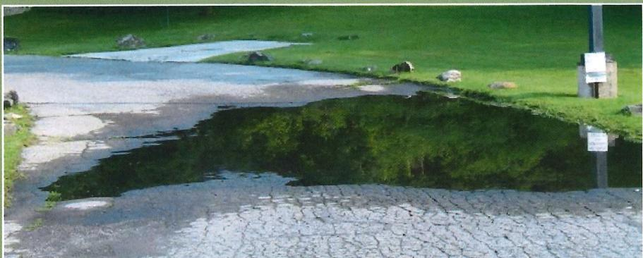
This condition is typically characterized by inadequate roadway cross slopes holding water on a roadway. This can also be contributed to improper shaping of the road; improper spacing and sizing of drainage inlets, and blocked culverts usually cause poor drainage.
