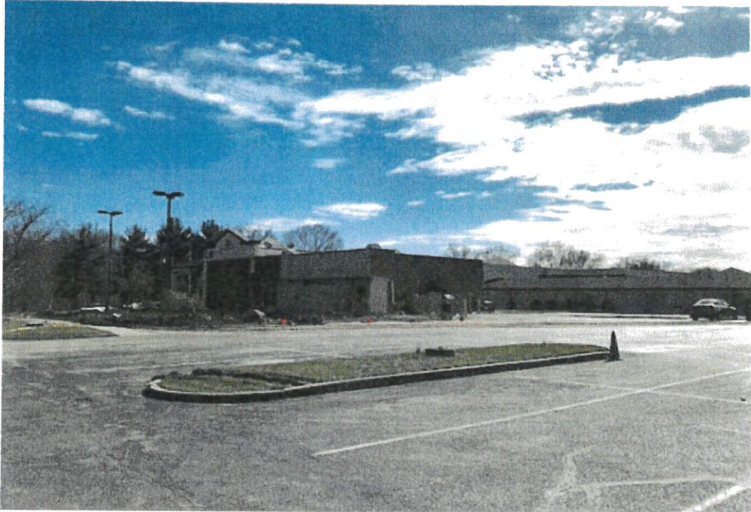
Photo 3. View of the front of the Red Roof Inn and the demolished Howard Johnson's Restaurant.
