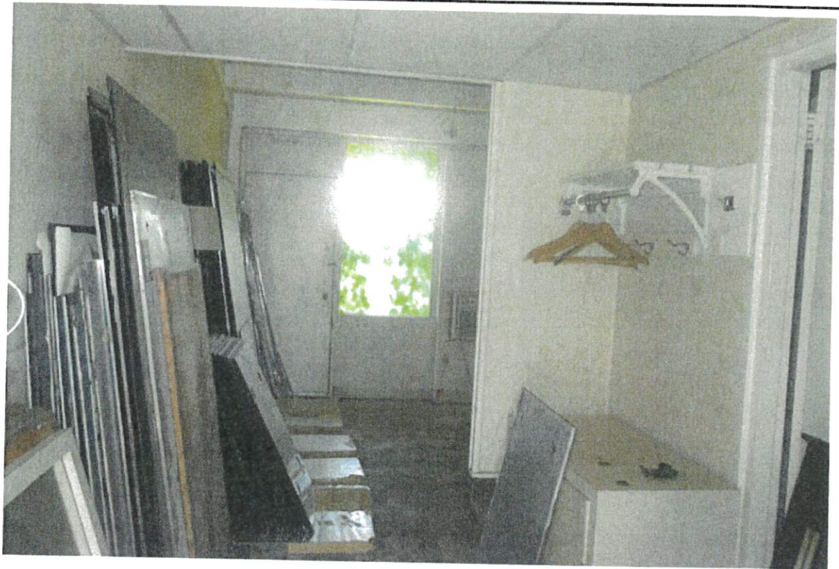
Figure 29: Interior view of a typical motel room in Building C.
