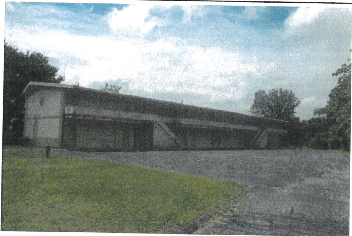
Figure 25: Looking at the front of the vacant former Howard Johnson's Motor Lodge motel building that is known as Building B.
