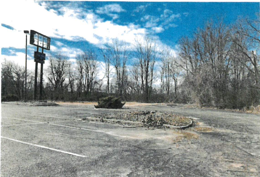
Photo 1. View of the northeastern side of the site where the Travel Agency and Howard Johnson's Motor Lodge office one stood.
