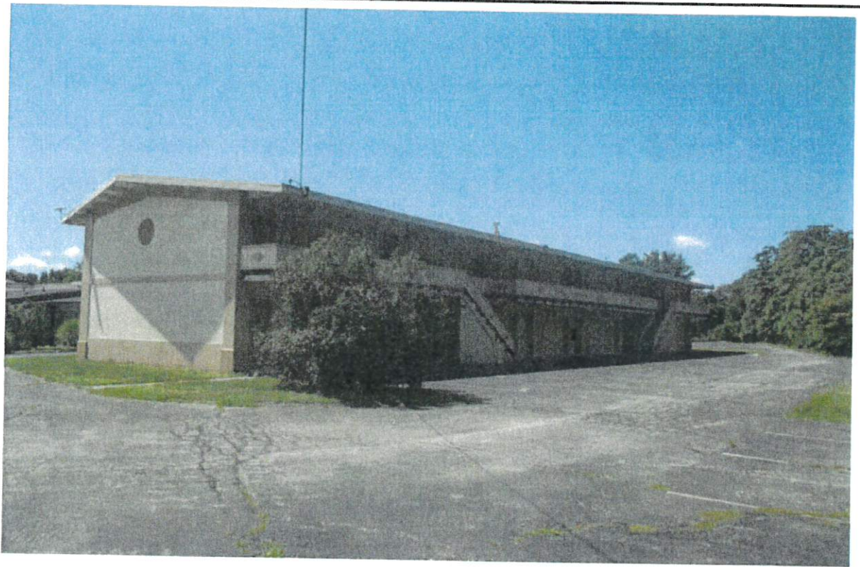
Figure 23: Looking at the front of the vacant former Howard Johnson's Motor Lodge motel building that is known as Building A.
