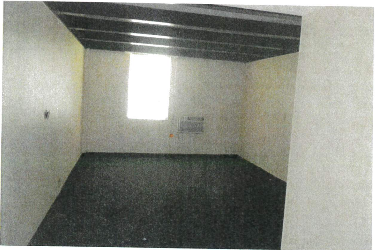
Figure 24: Interior view of a typical motel room in Building A.
