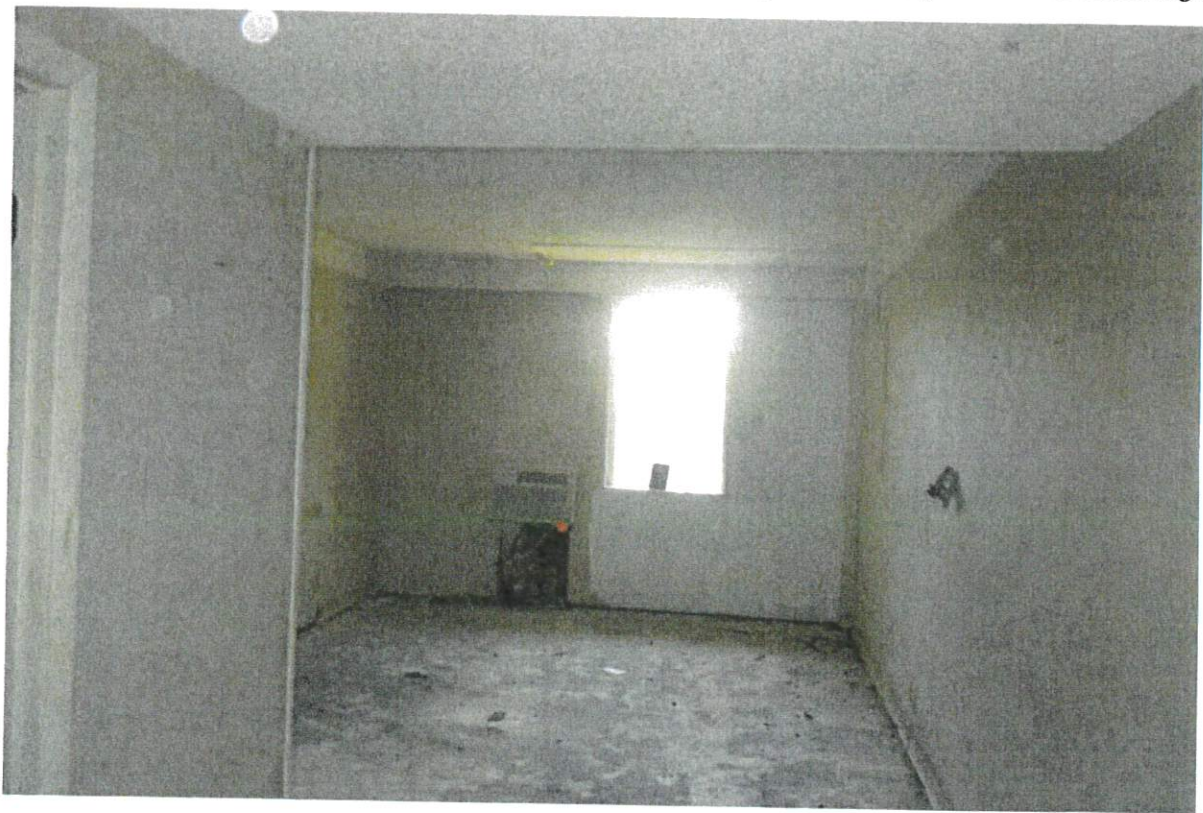
Figure 26: Interior view of a typical motel room in Building B.
