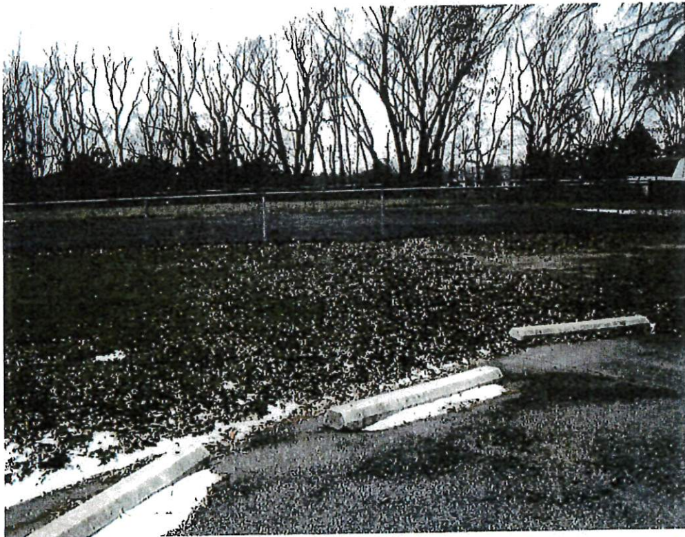
Existing Deteriorated Court & Inadequate Fencing
